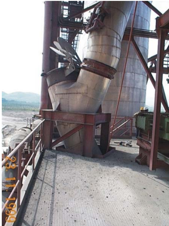
Thorwestern Vent's "vent # 1 + vent # 2" concept's self-reclosing vent # 1 (explosion door)
