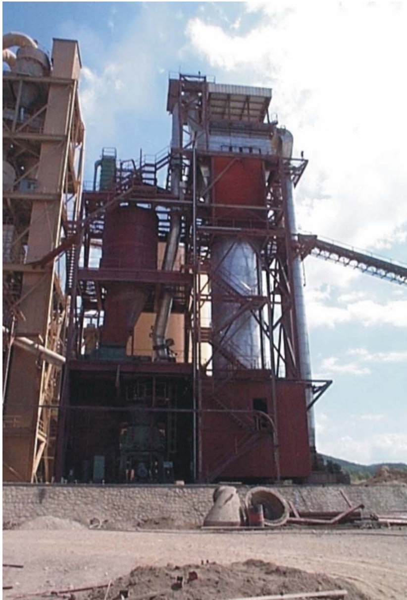
Typical vertical roller mill coal grinding system with long mill-to-dust separator duct, illustrating considerable overall height of system
