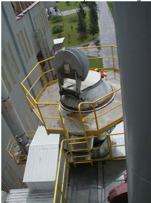
Thorwestern Vent's "vent # 1 + vent # 2" concept's self-reclosing vent # 2 (explosion diverter)
